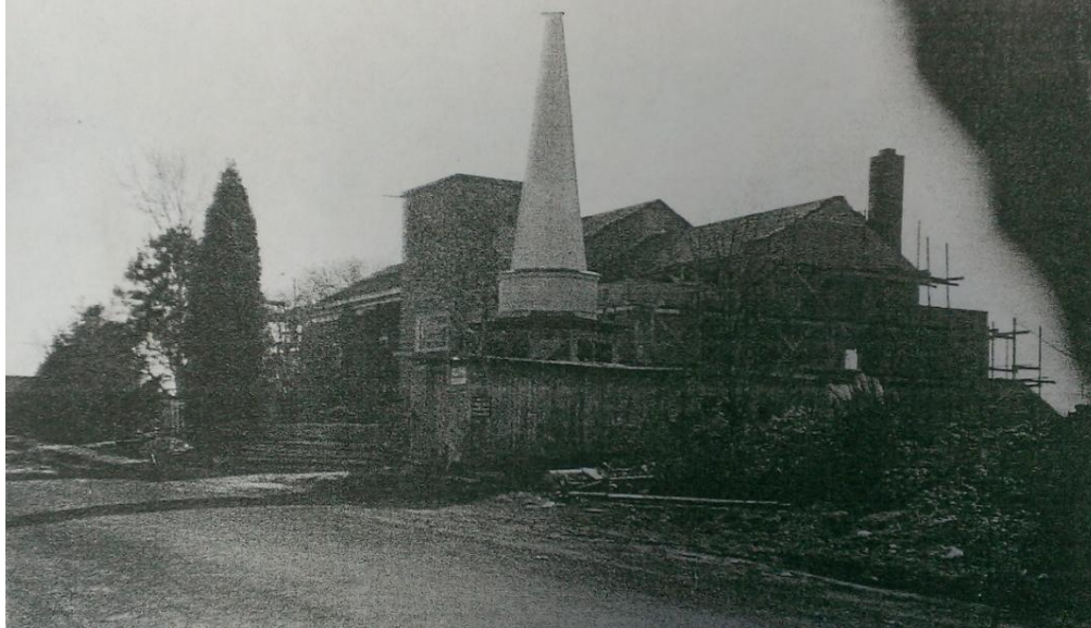
Figure 32: View of north and east elevations of Arlington Presbyterian Church, showing the raising of the lantern and spire and other construction efforts, ca. 1950. Note the gable addition to the original church.
