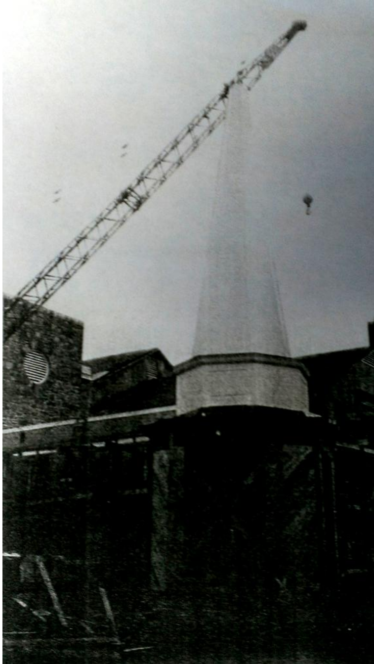
Figure 31: View of north and east elevations of Arlington Presbyterian Church, showing the raising of the lantern and spire, ca. 1950.
