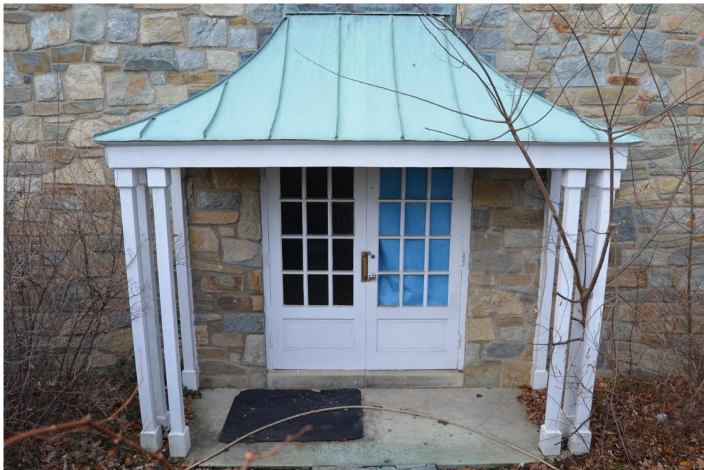
Figure 8: Double-leaf wood door sheltered by a flared standing seam metal roof supported by wood posts. The entrance is located on the east elevation of the 1961 gable roof addition.
