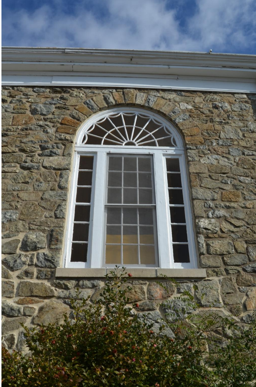
Figure 14: Typical nine-over-nine, double-hung, wood-sash window with six-light sidelights and decorative fanlight.
