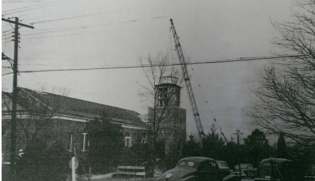
Figure 34: View of south and east elevations of Arlington Presbyterian Church, showing the lowering of the lantern and spire on the tower, ca. 1950. Source: Arlington Presbyterian Church Archives.
