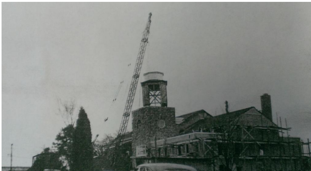
Figure 33: View of north and east elevations of Arlington Presbyterian Church, showing the raising of the lantern and spire and other construction efforts, ca. 1950.
